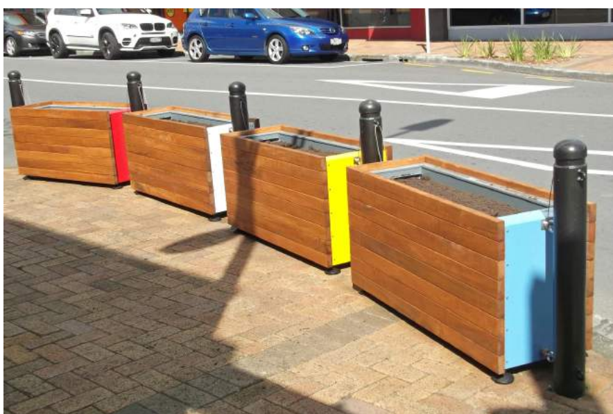
The planters at left are located on Main Street, Upper Hutt, made using vitex hardwood and sheet-steel on a heavy-duty galvanised mild-steel frame.
