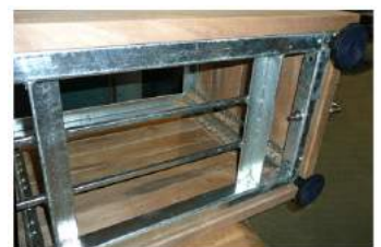
The planters at left are located on Main Street, Upper Hutt, made using vitex hardwood and sheet-steel on a heavy-duty galvanised mild-steel frame.
